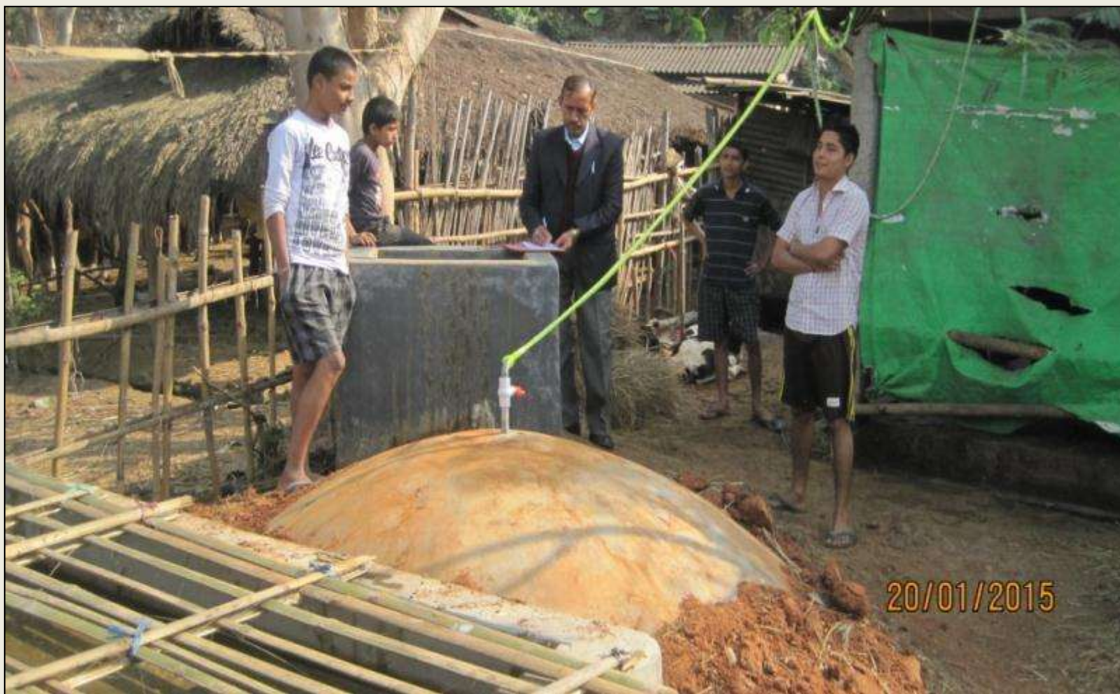
A 3 M 3 Deenbandhu Biogas Plant under Construction in Jan 2015 at village –Panikhet, District - Kamrup, Assam
