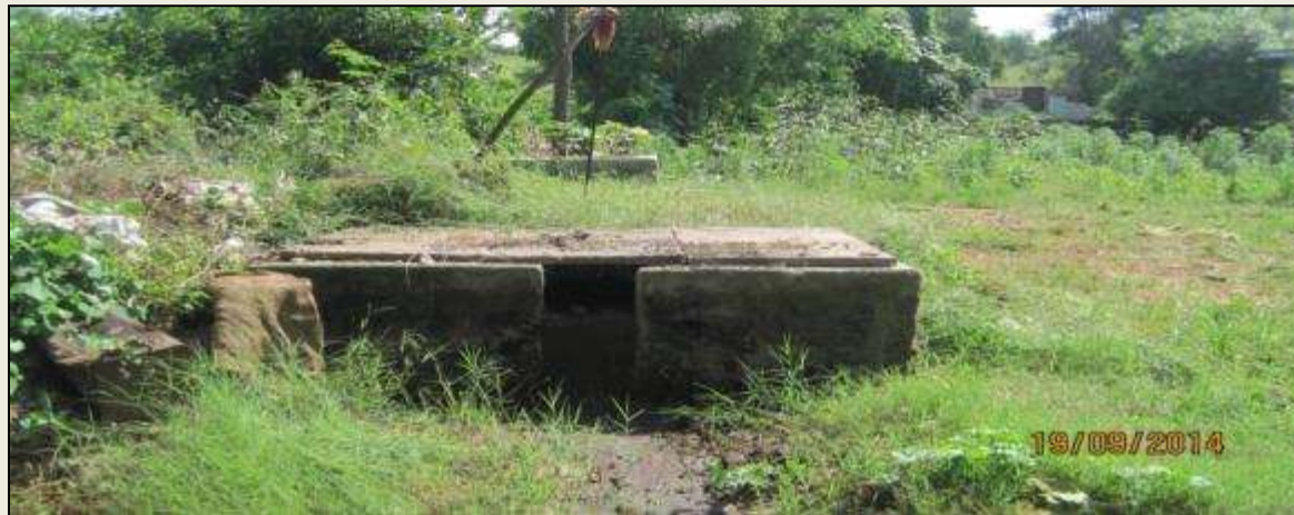
A 2 M 3 Solid-state Deenbandhu Biogas Plant at Kherwara, District- Udaipur, Rajasthan. Despite of Beneficiary having LPG connection, using Biogas as predominant fuel for cooking.
